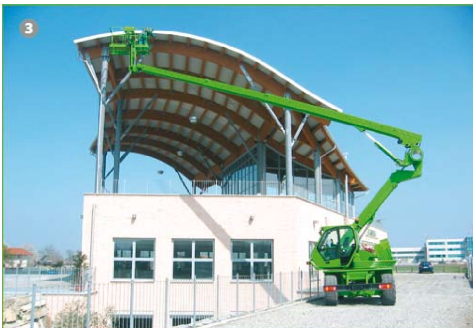
3 And then work in complete safety at up to 30m high
